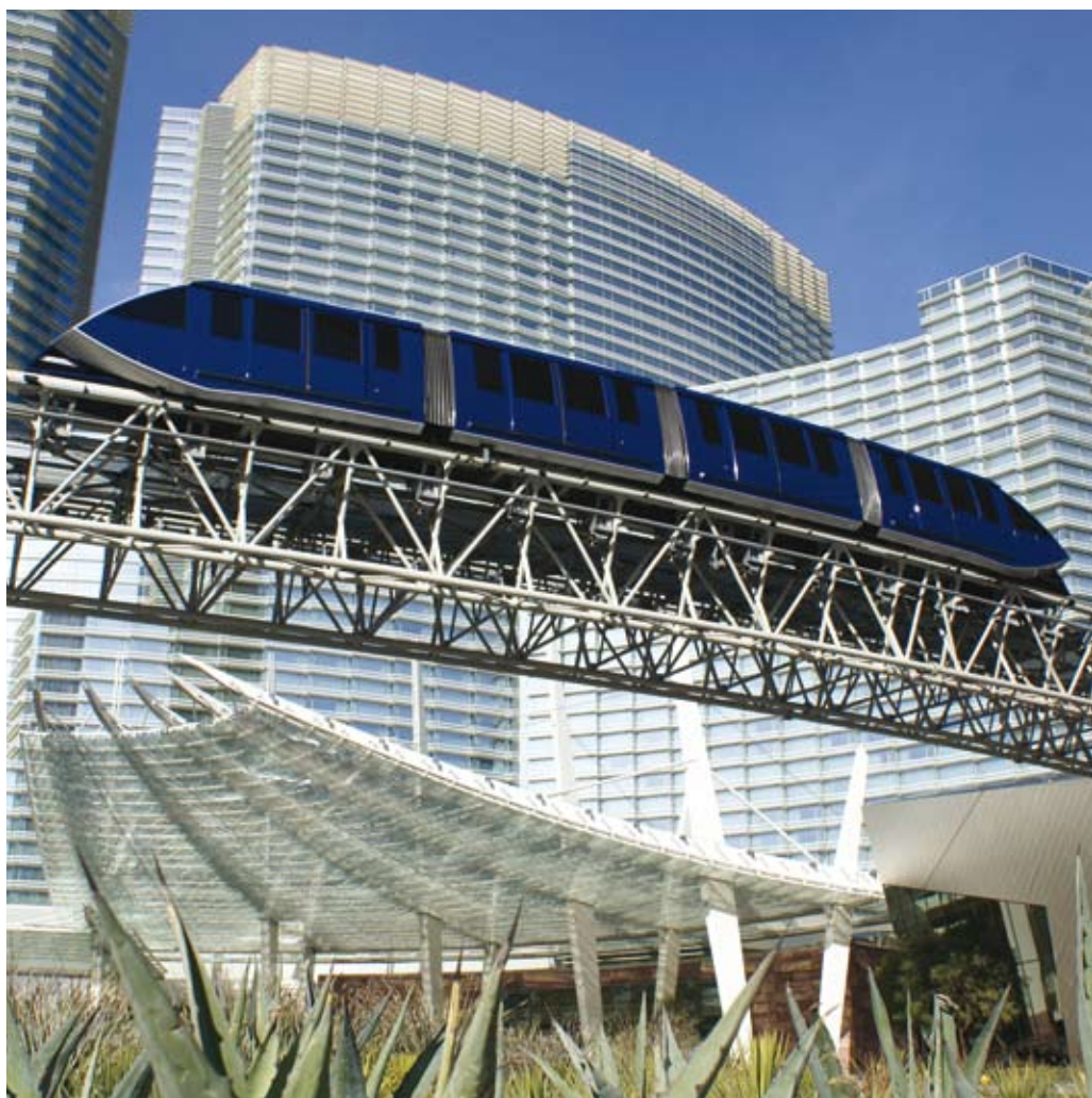
Fig. 1: Rope-propelled Automated People Mover in Las Vegas, Nevada
